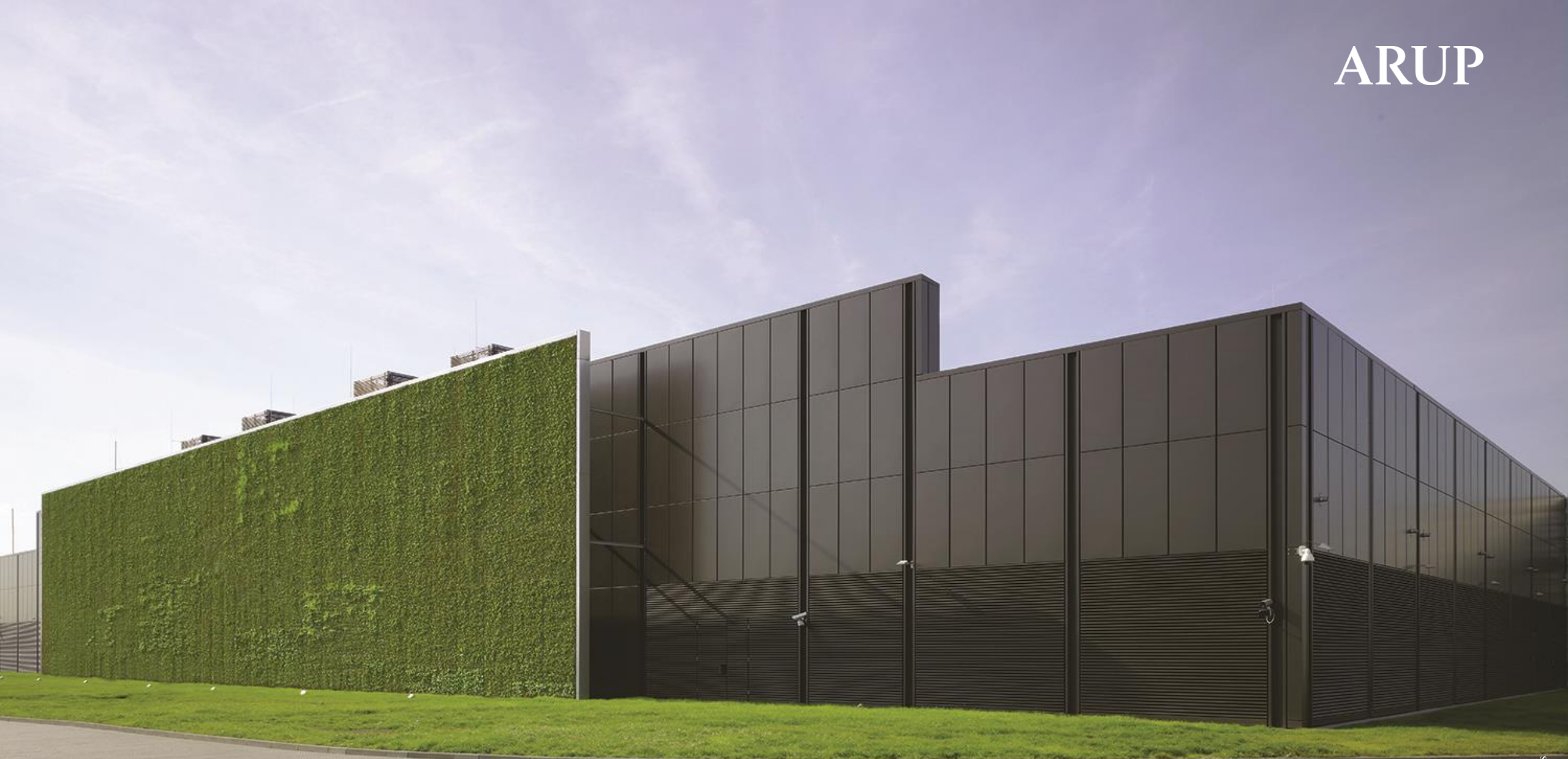
Citibank Data Center, Frankfurt am Main
